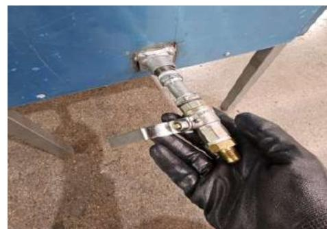
**2** Connect the shut-off valve and terminal nipple to the fryer
