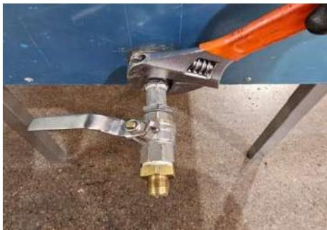
**3** Tighten the shut-off valve, ensuring it is securely fastened
