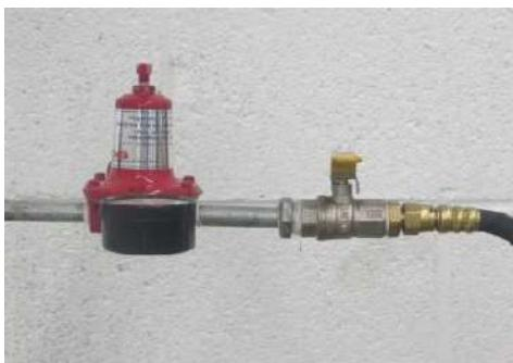
**1** Connect to the gas supply using a high-pressure regulator
