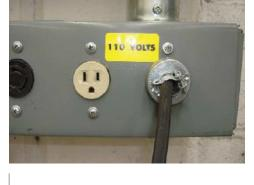
2 Connect extruder cable to 110v outlet
