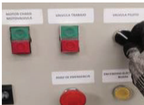
I Turn the pilot valve knob (OFF), the indicator will turn off.
