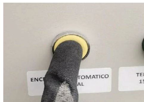
B Activate the power button general automatic for 5 seconds.
