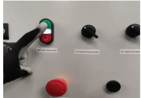
D Main motors will start and the indicator will illuminate (green light)
