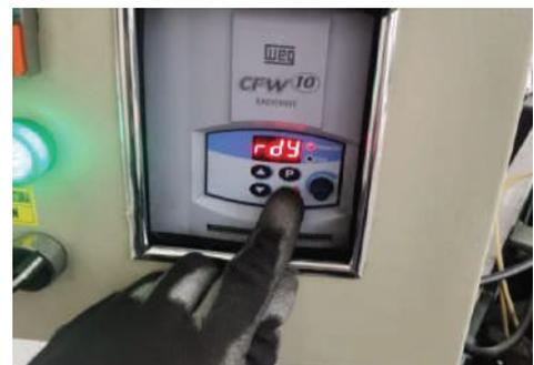
**6** Press the ON button (green) of the variable speed drive to turn on the main motor.
